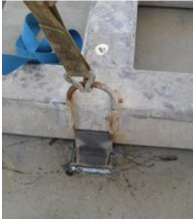
10.10 Sample of cradle positioning welds.
