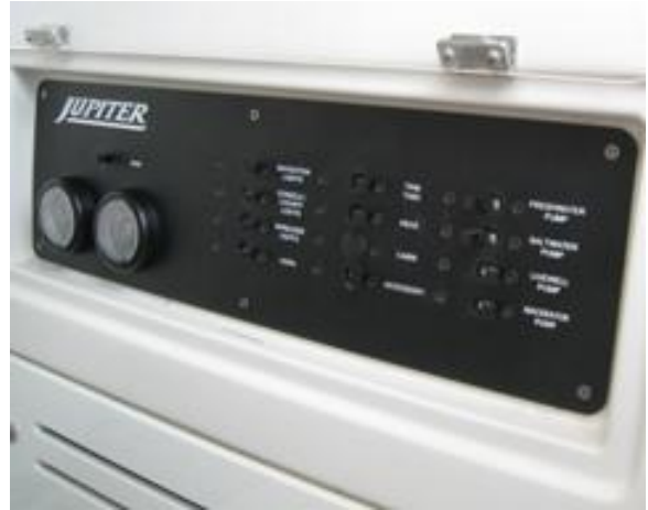
DC control panel mounted in head
