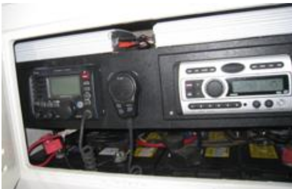
Radio gear & batteries mounted in head
