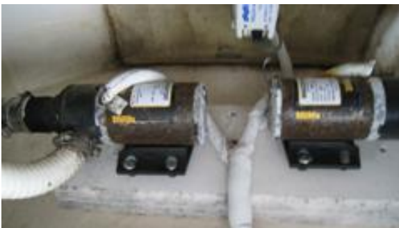
Keep an eye on these motors, lots of corrosion.
